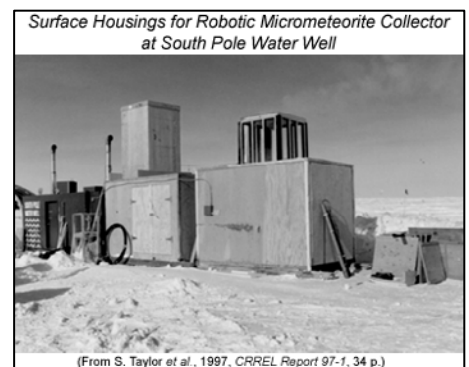
These shelters (winch room and laboratory) at the South Pole Water Well house the tower assembly, winch and cable system, video equipment, and control equipment needed to support the remote-controlled collector
