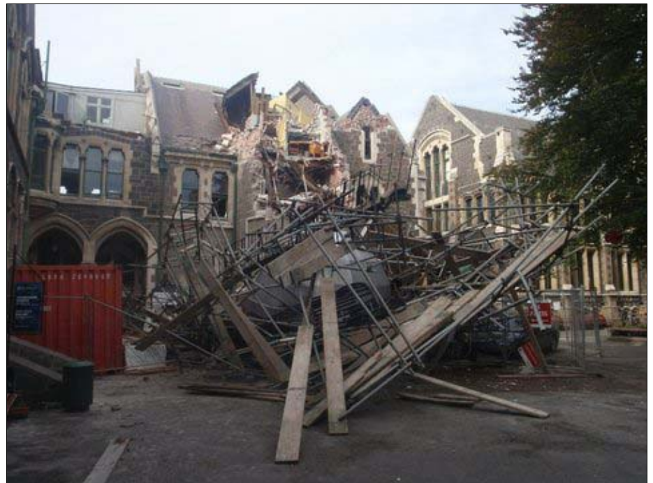
The ruined Townsend Observatory at the Arts Centre in Canterbury
