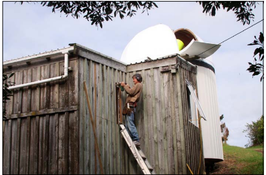
Peter McLeod installing windows at the Kumeu observatory
